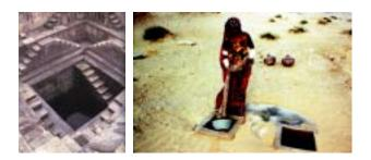
Using peoplres knowlegde, in 1986 the Barefoot College constructed a 400,000 litre underground rain water harvesting tank on the on the campus. It is fed by pipes from roof tops and ledges and has an overflow into an open well. The impact of this exercise has been far reaching.
